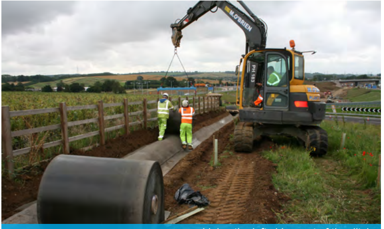
Lining the left side crest of the ditch
