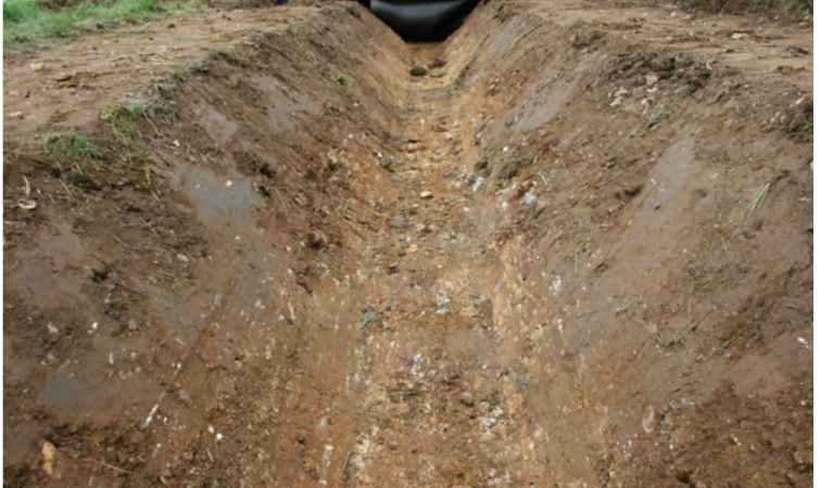
Graded ditch section with vegetation removed.
