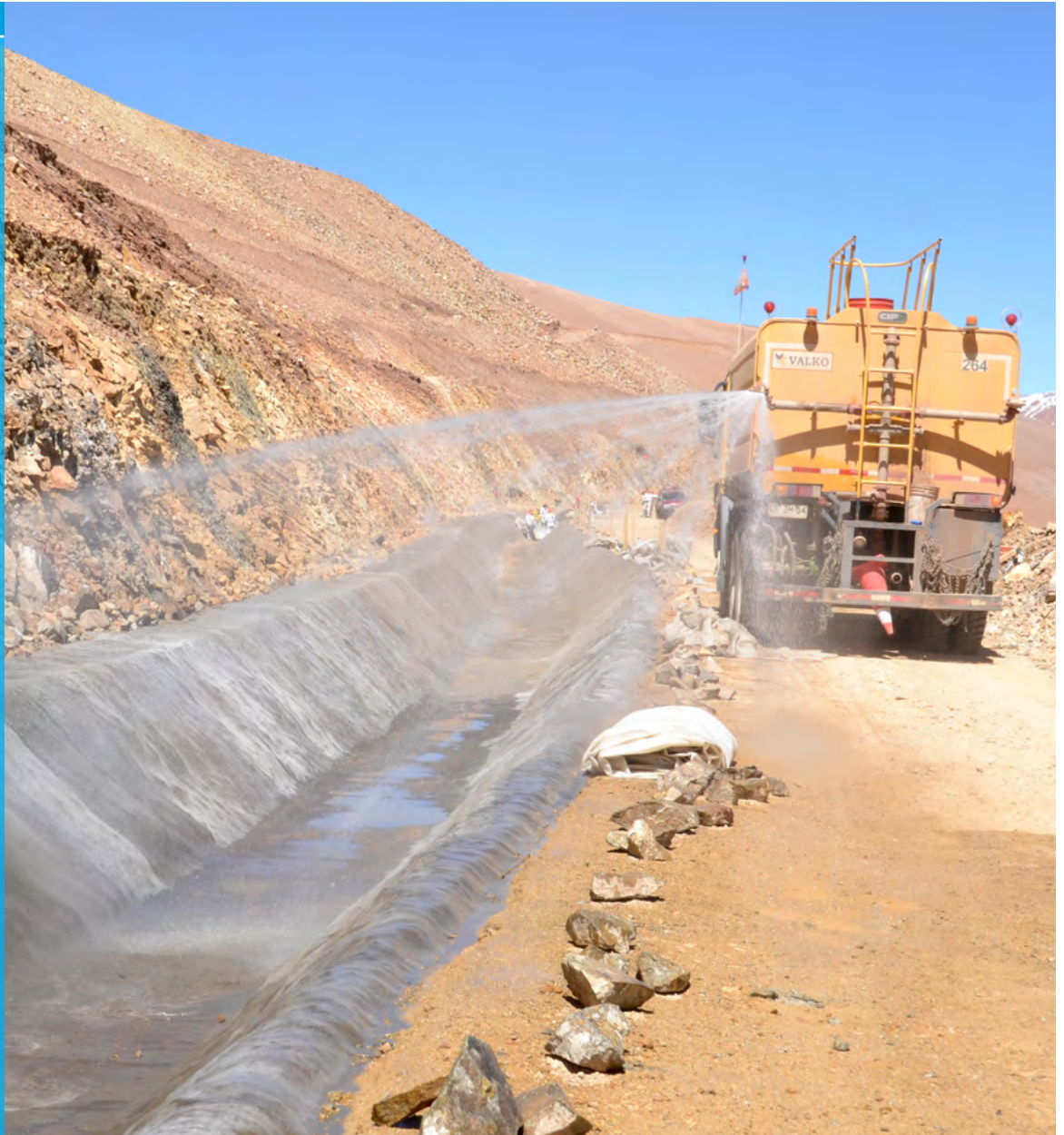
Section of CC-lined ditch undergoing hydration
