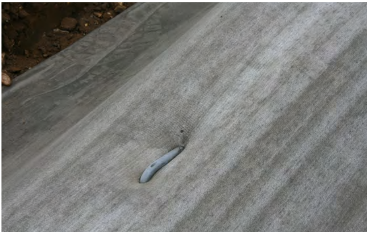
CC was secured with steel ground pegs at 2m intervals.
