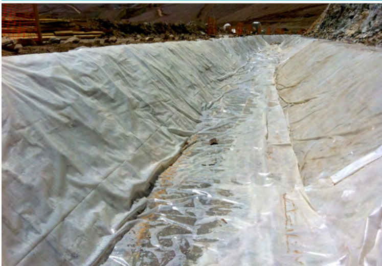
Hydrated CC covered with plastic sheeting to protect from low temperatures
