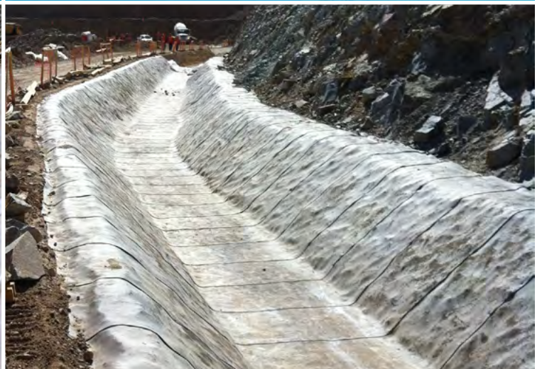
Completed lined section of ditch
