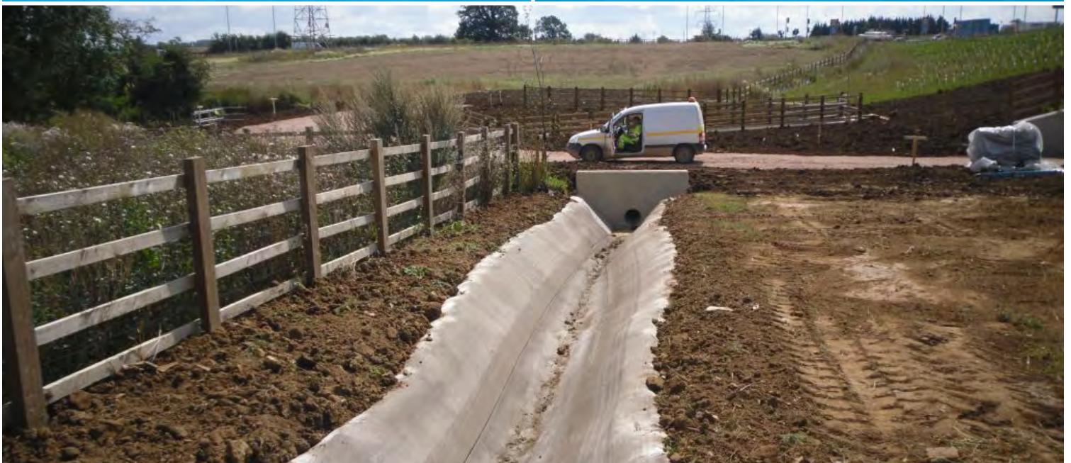
Completed CC ditch section terminating in concrete culvert.
