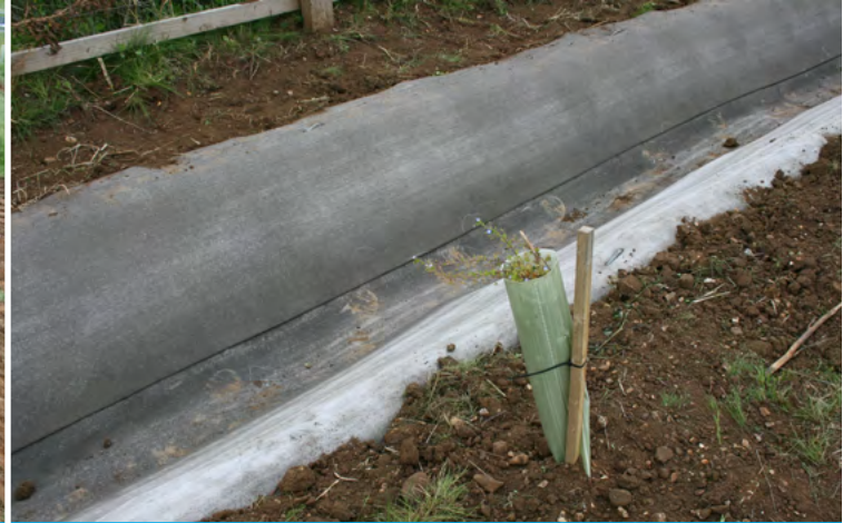
Detail showing overlap between longitudinal CC layers
