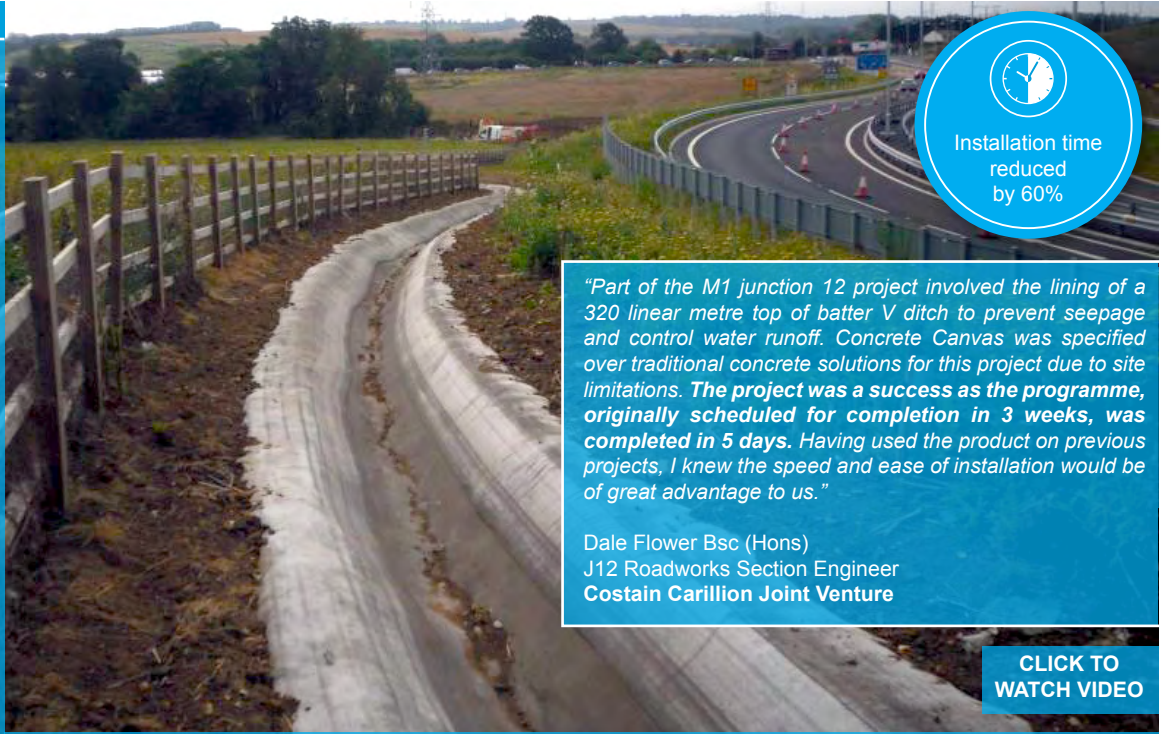
Completed lined ditch section
