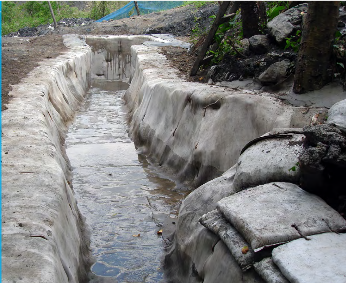
Completed CC lined trap
