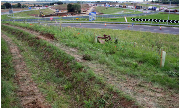
Batter prior to ditch excavation.
