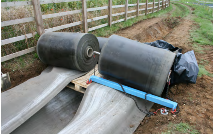
CC Bulk rolls arranged for installing three longitudinal layers
