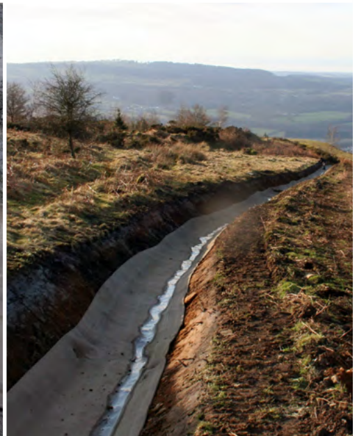
Completed CC lined channel
