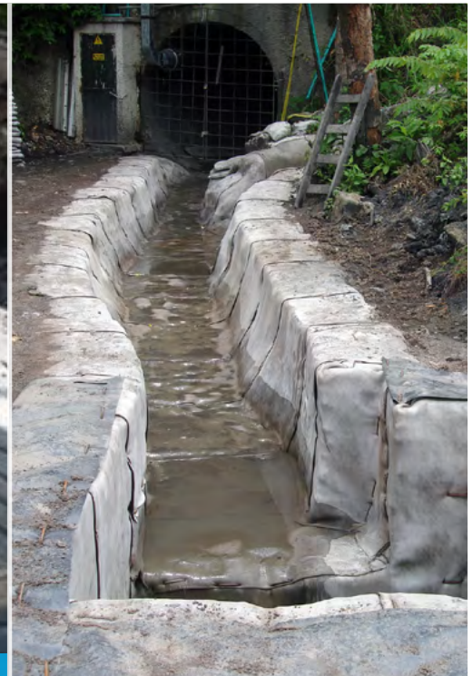
CC fixed with re-bar fixings
