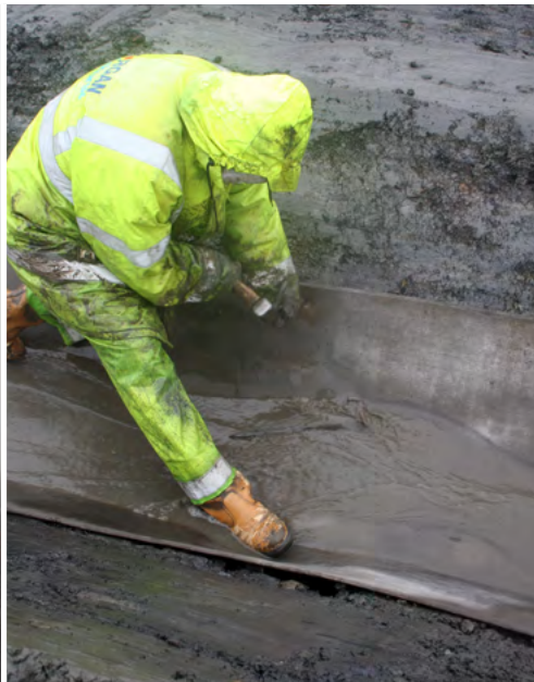
CC secured to substrate with pegs
