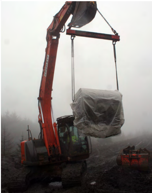
CC bulk roll transported to site
