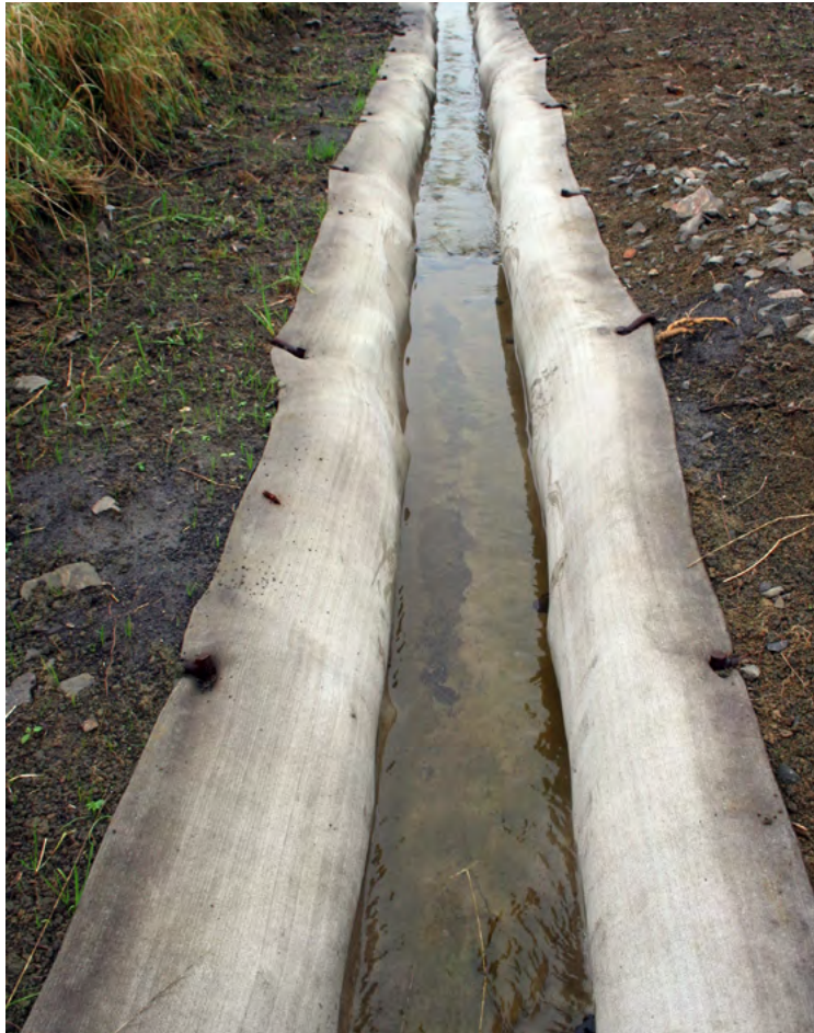
Completed ditch with water flow
