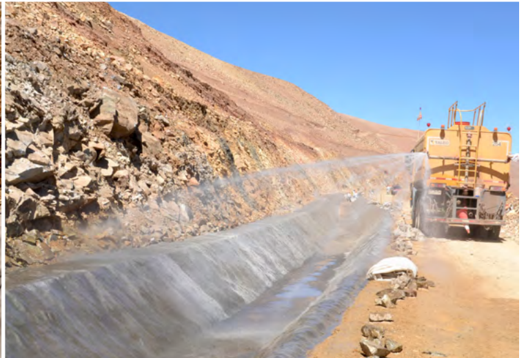
Water/accelerant mix dispensed from water tanker during hydration
