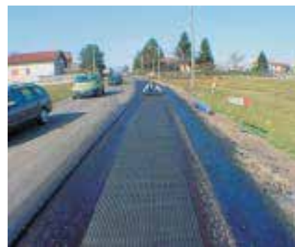
Posa in opera del geocomposito Armapal
